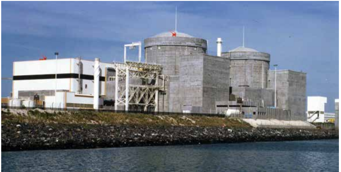
Koeberg power station
