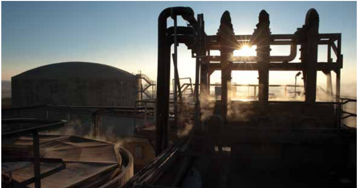
eMalabeni Water Reclamation Plant
