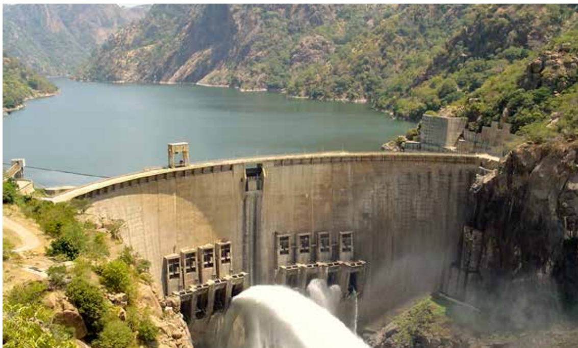
Cahora Bassa Dam, Mozambique
